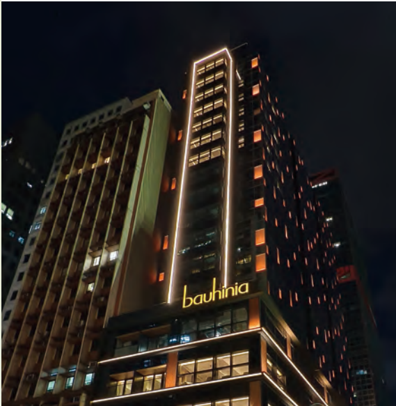
The Bauhinia Hotel (Central) – BIPV System
